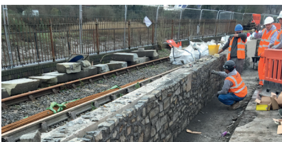
Metrobus flood wall under construction, Cumberland Road
