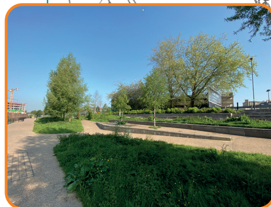
Submergible path and park, Bath Quays
