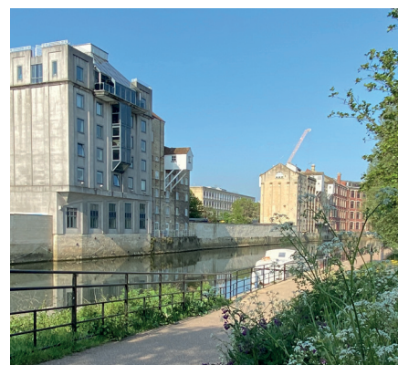
Flood defence combined with development at Bath Quays
