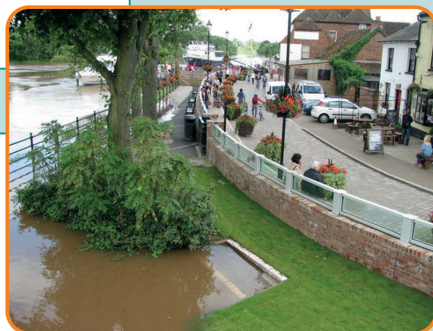
Glass panels as part of flood defences, Upton-upon-Severn, Warwickshire
